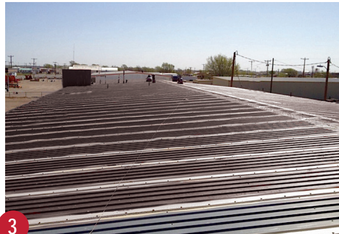
Metal roof after application of Spunflex® fabric and Rapid Roof® base coat to the seams along with Kwik Kaulk® sealant application to the fasteners.
