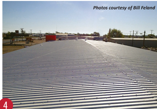
Metal roof after Rapid Roof® acrylic top-coat.
