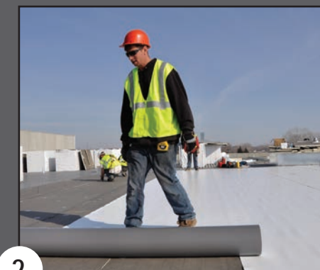
2 Apply membrane, overlapping seams in the direction of water run-off.
